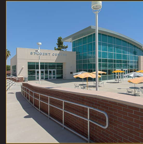
South Facade Opens to Quad
